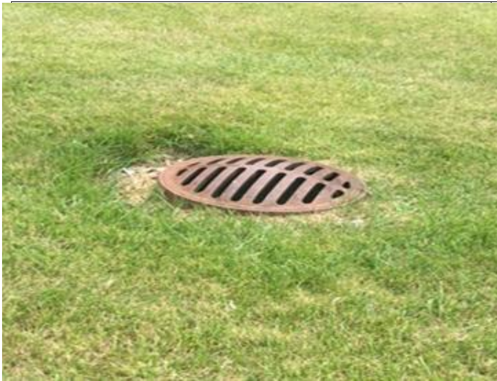
Fill around existing Catch Basin in Nutmeg Park
