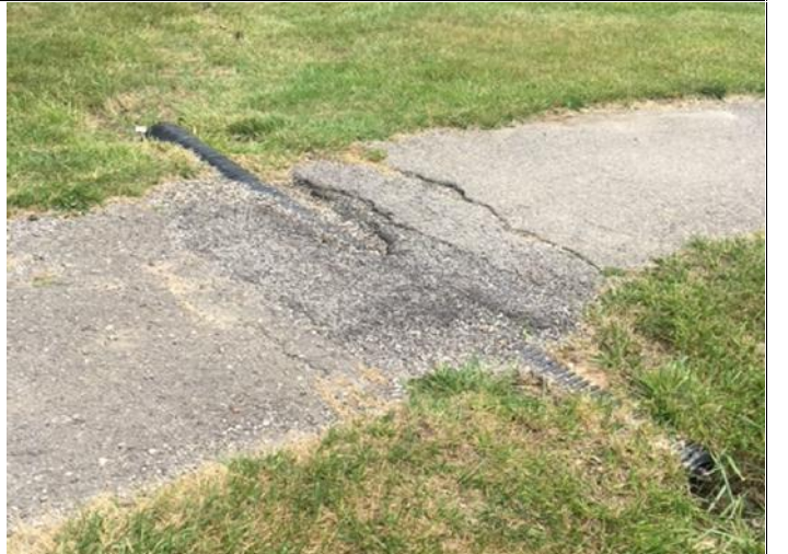
Replace Culvert & Repair Bituminous Pathway
