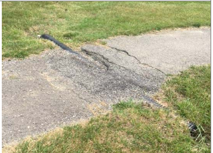
Replace Culvert & Repair Bituminous Pathway
