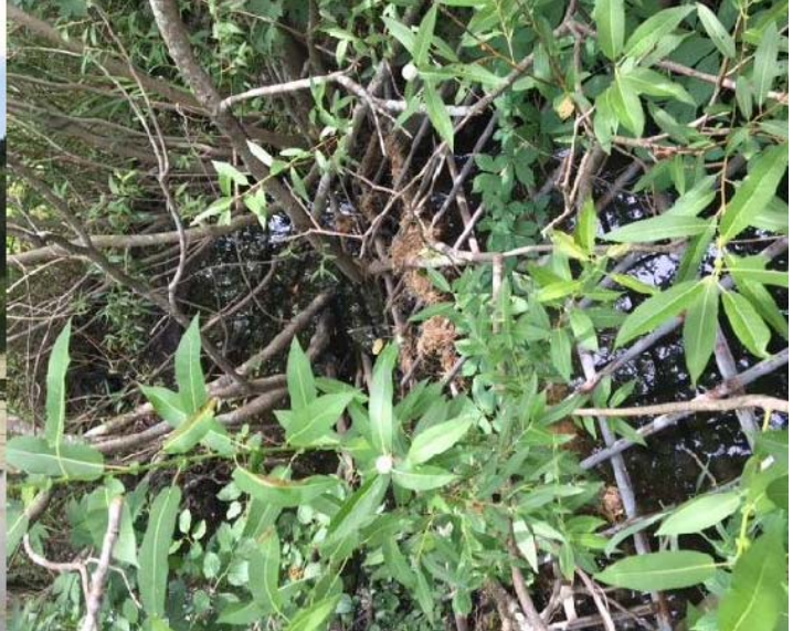
Remove Brush from Detention Basin Inlet Sewer
