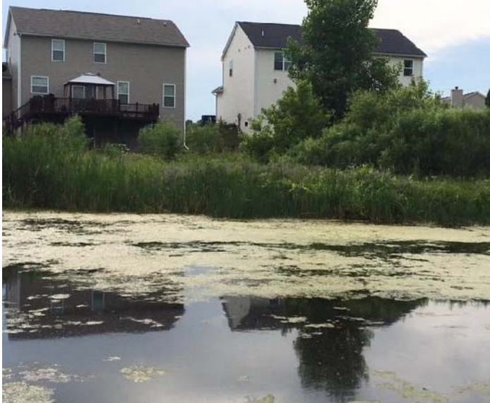
Remove Brush from Detention Basin Inlet Sewer
